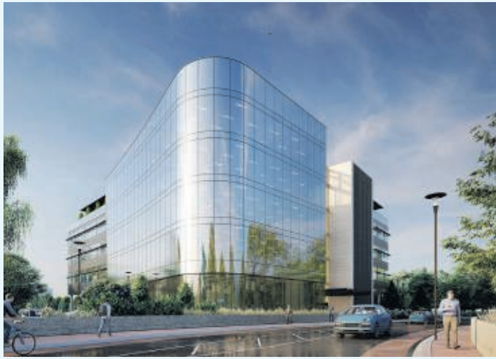
Second phase to begin at South County Business Park, Leopardstown
